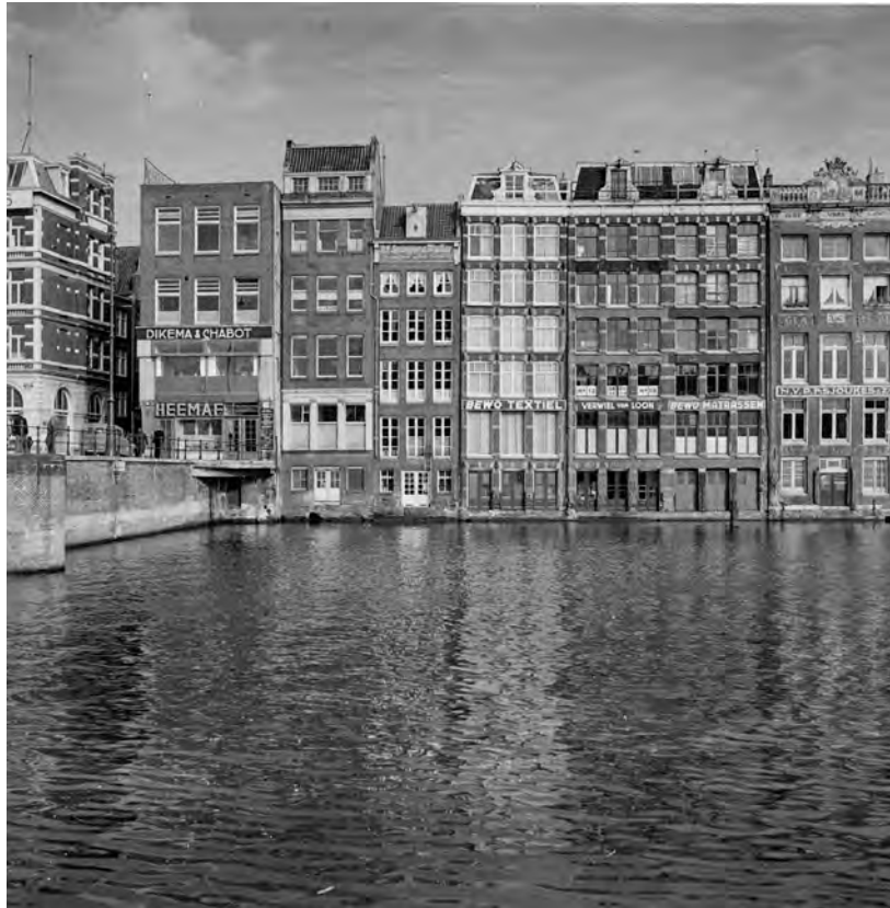
AMSTERDAM. Old houses. Image: Roberto Pane, end of the 1940s (AFRP, OLA.N.4).
