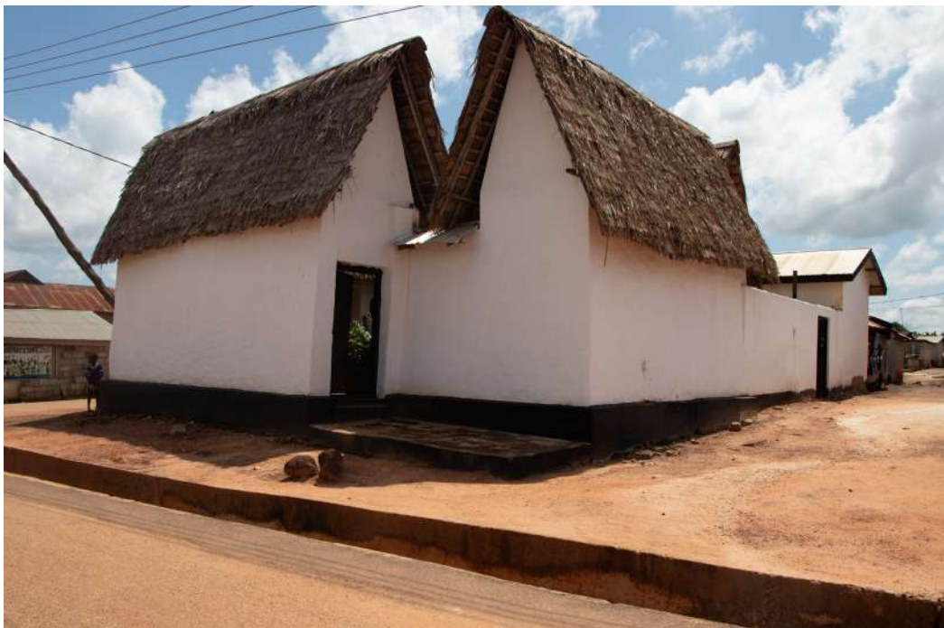
Figures 3.3 Beasease Asante Traditional Building (Source: Chris Wetcher, 2019)
