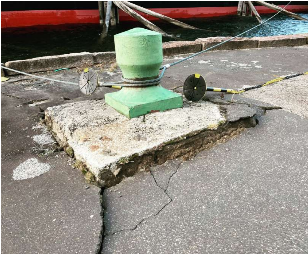
Figure 9.5 Damage to the mooring structures of the railway ferries at the wharf facility of Mæl, a consequence of the extreme weather events of 2021. (Source: Norsk Industriarbeidermuseum)
