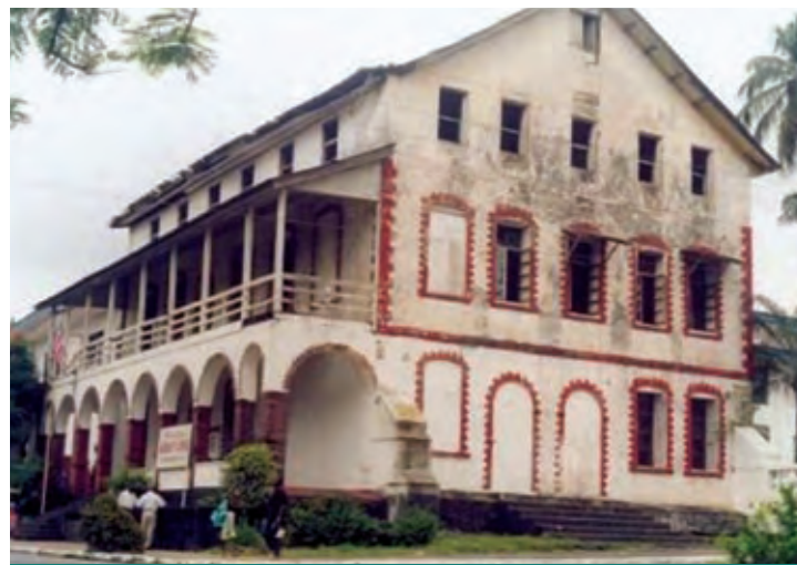
FIGURE 65 The National Museum of Liberia, after shelling during the war in the 1990s.
