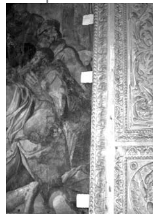
17 Church of St. Eligio: Salts analysis on mural painting colour print on inside back cover
