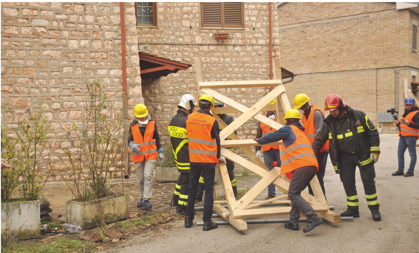
Participants during a shoring exercise with the Vigili del Fuoco in Norcia, Italy, 2019 © ICCROM
