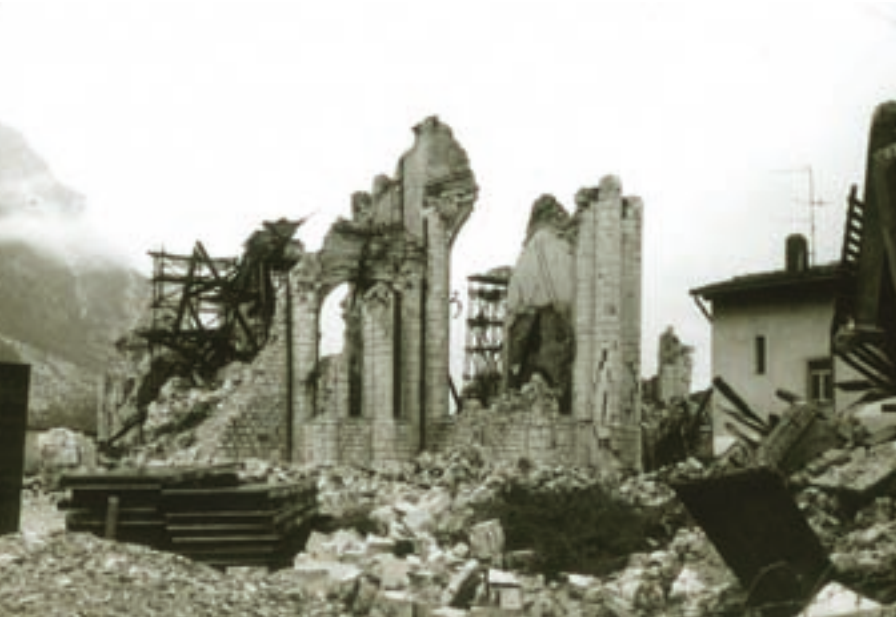
FIGURE 4-27 Friuli earthquake, Venzone cathedral, photogrammetric record by ICCROM-Austrian team after second quake
