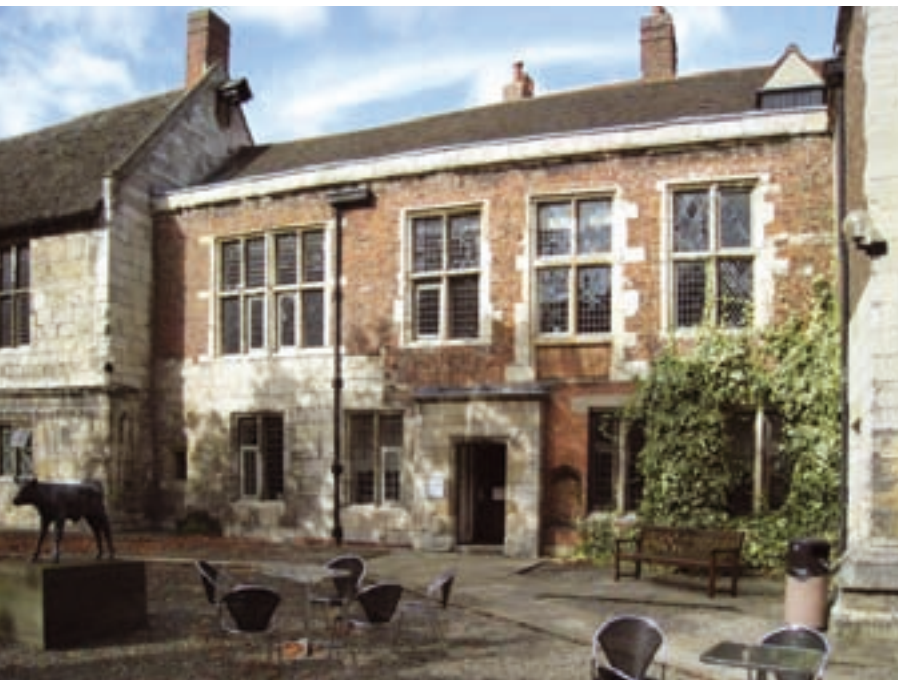
FIGURE 5-12 Inner courtyard of the historic King's Manor in York, home of the Institute of Advanced Architectural Studies (IoAAS) of the University of York, with which ICCROM signed an MoU for exchanges in conservation training
