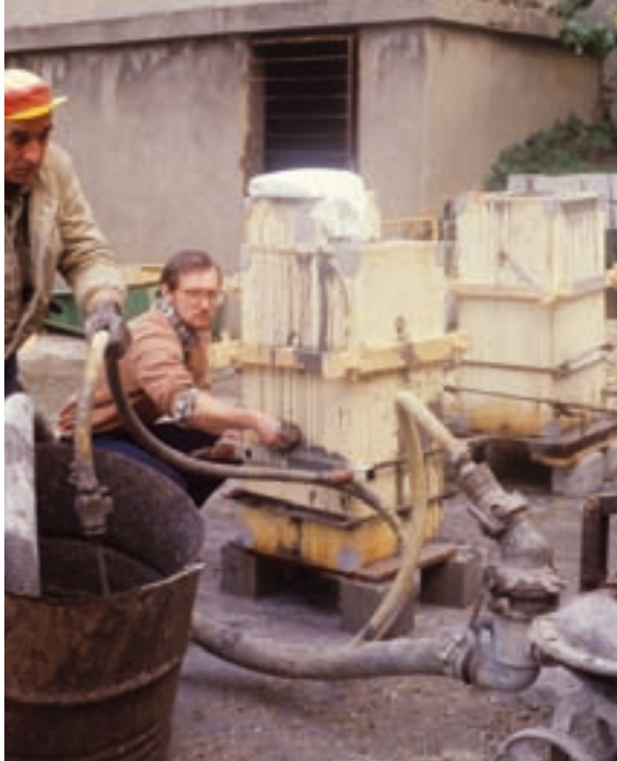
FIGURE 5-34 Mortar mixture being prepared by a team directed by G. Torraca (in picture: Jef Malliet)
